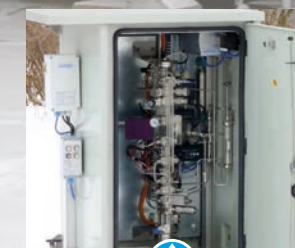
Compact field enclosure with three separate analyzers and sample conditioning (from Astute).
