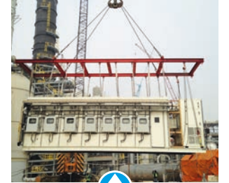
INTERTEC's turnkey service can greatly simplify projects - in this case an analyzer shelter for a Saudi Arabian plant was designed, manufactured and fully assembled at INTERTEC's factory - before shipping in one piece to the plant for rapid installation.
