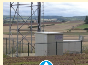
Lightweight cabinets and shelters for mobile communication sites, simplifying transportation to remote or difficult locations, such as by helicopter to building rooftop installations.
