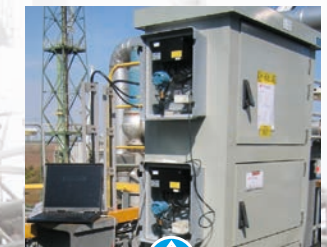
Analzers are critical to oil and gas plants - and many new forms of smaller and online analyzers are being installed - often in inaccessible areas. Custom enclosures simplify such applications. This small-footprint and light 'hot box' maintains 140°C and was designed for easy retrofit on a process column.
