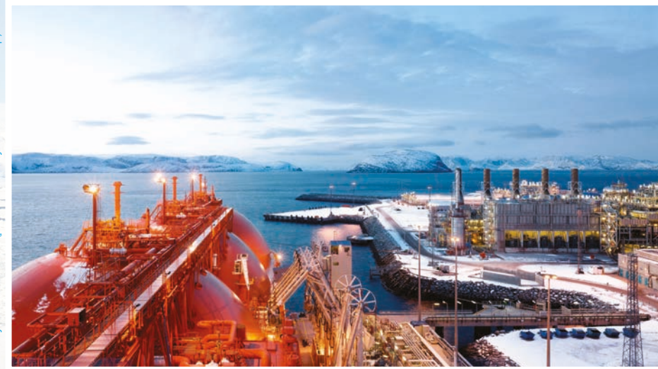
Melkoya LNG terminal (photo courtesy of The Linde Group).
