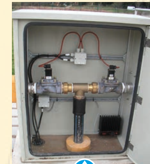
Sandwich construction cabinets with thick embedded insulation minimize heat losses - requiring only a small heater to protect against freezing.
