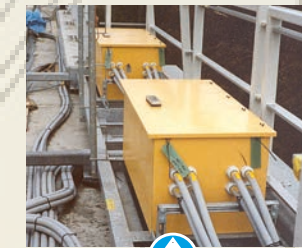
GRP cabinets for high current switches feature a metal-free exterior surface to eliminate eddy current losses.
