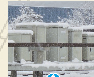
Sandwich construction with thick foam insulation provides stable operating environments for these above-ground metro equipment cabinets.
